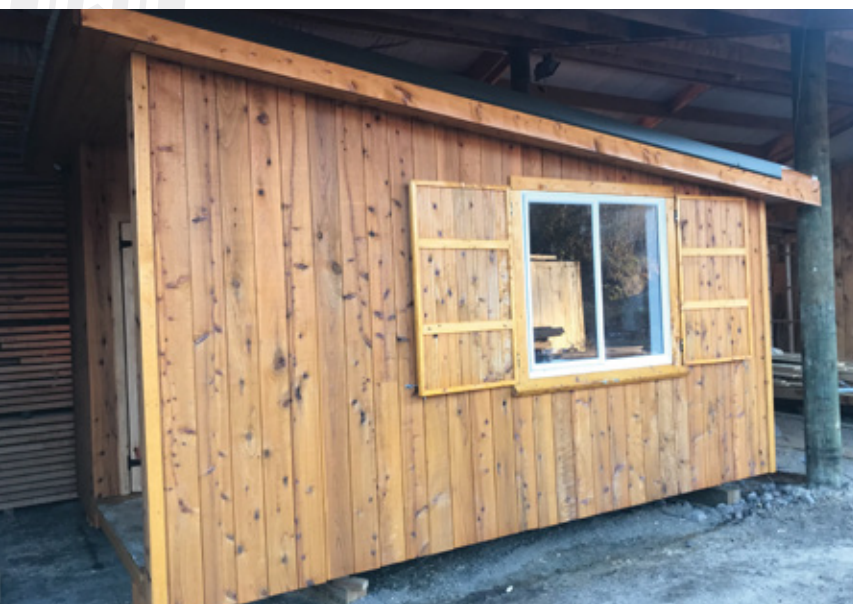
Above right: Cryptomeria japonica timber. Below: Cabin with C. japonica shiplap cladding.
