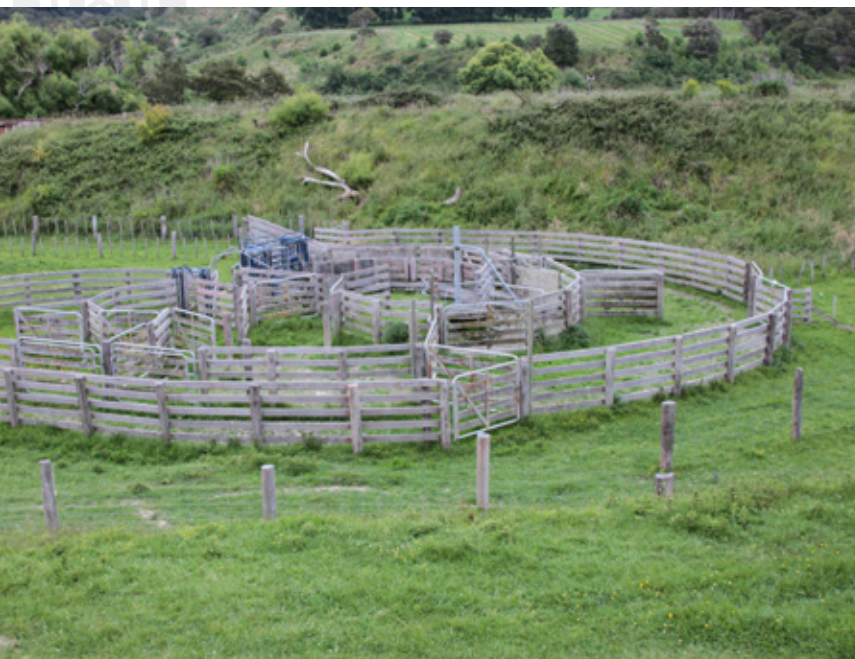
Above: An NZDFI peeling trial using mixed species of durable eucalypts to produce naturally durable posts. Below: Cattle yards constructed with locally grown E. globoidea , Gisborne.
